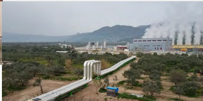
POWER performed the detailed design for the Kizildere Geothermal Power Plant in Turkey.
